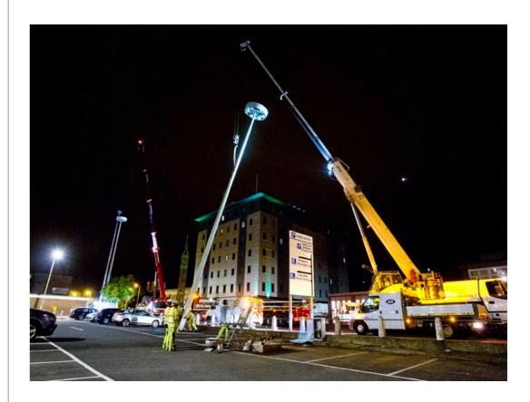
Stevenage High Mast Lighting Maintenace Work
